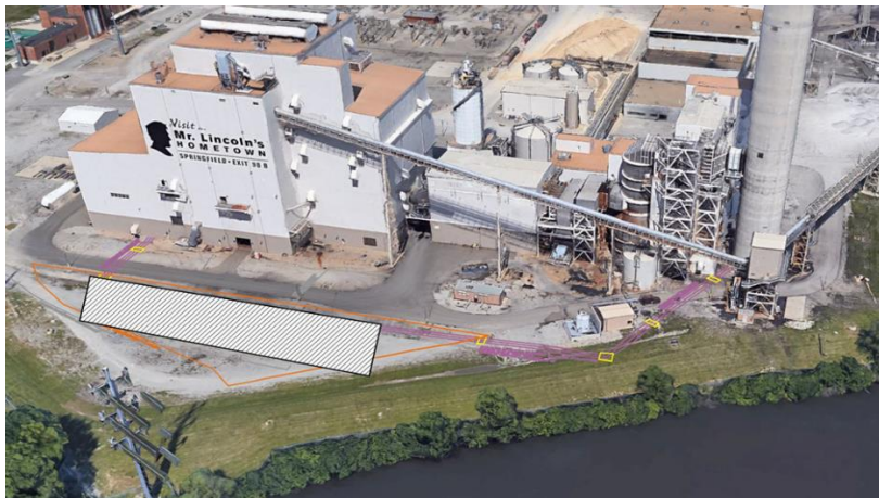
Fig. 4. Dallman #4 unit at CWLP with proposed capture plant location (hatched rectangle); purple lines - utilities; yellow boxes - duct work supports.
